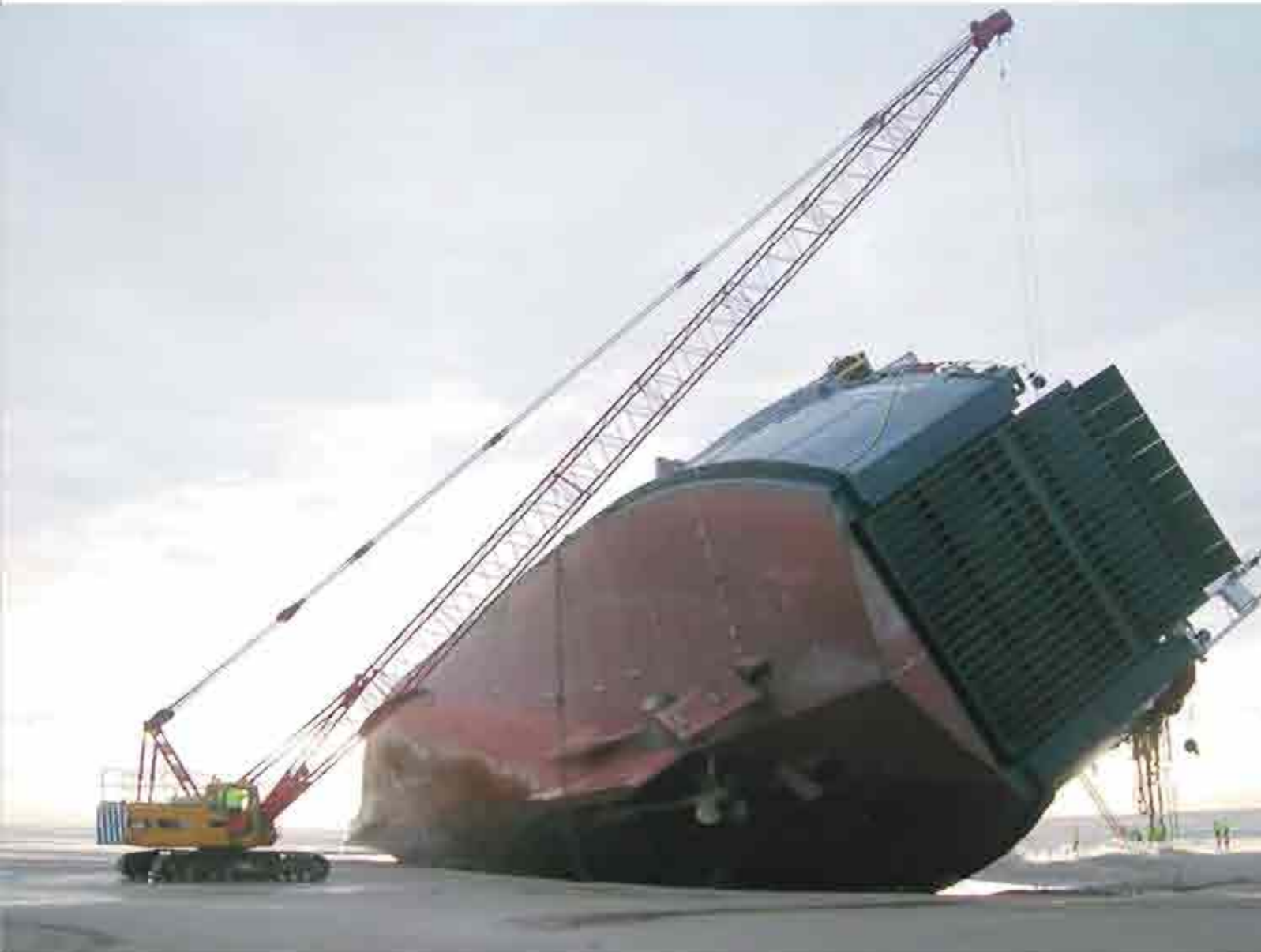
One of the first SANY HG32C Hydraulic Crawler Cranes was used to keep a ship steady during a refloating operation after it ran aground off Blackpool on England's Irish
